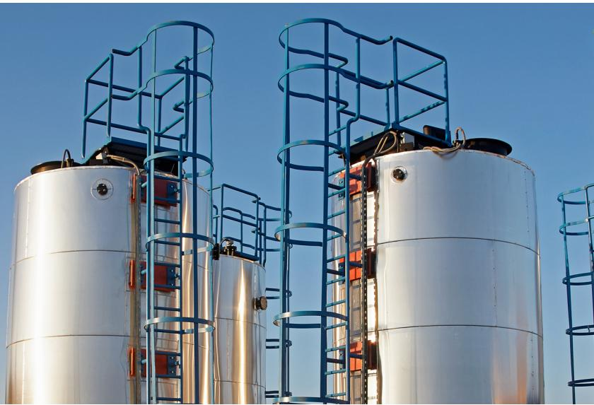
LLT100 level measurements with use of laser technology in mixer chemical tanks
