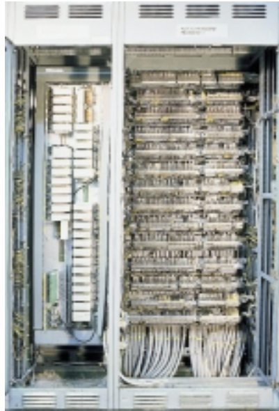
The new controller is quickly connected, using existing process cabling, by bus communication to the Advant Controller.
