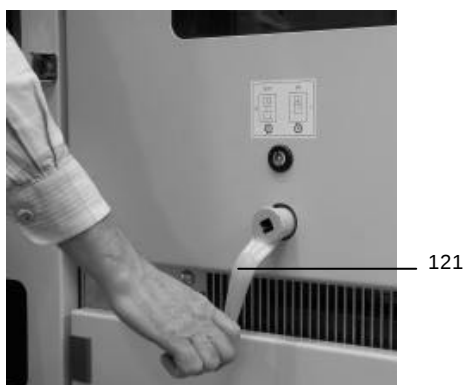
Figure 6/3: Movement of the withdrawable part between the test/disconnected position and the service position, clockwise up to the stop to the service position and anti-clockwise for the test/disconnected position
