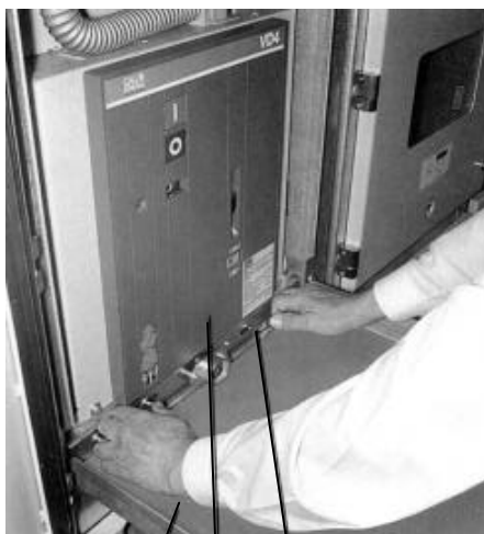
Figure 6/5: Service truck engaged with the switchgear panel. Withdrawable part released for withdrawal with the handles slid inwards
