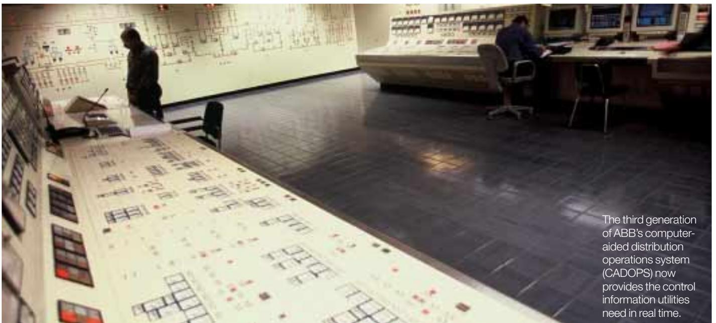
The third generation of ABB's computer-aided distribution operations system (CADOPS) now provides the control information utilities need in real time.
