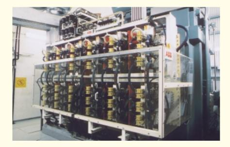
ity addition, is powered by a 135-kA, 770-V DC facility. ABB Industrie AG of Switzerland supplied the electrical equipment, including four single-phase main transformers, 220-kV, 33-kV and 21-kV switchgear, a thyristor-controlled rectifier station, reactive power compensating plant and the process control system. The latter system ensures efficient operation, plus high control response and accuracy.
