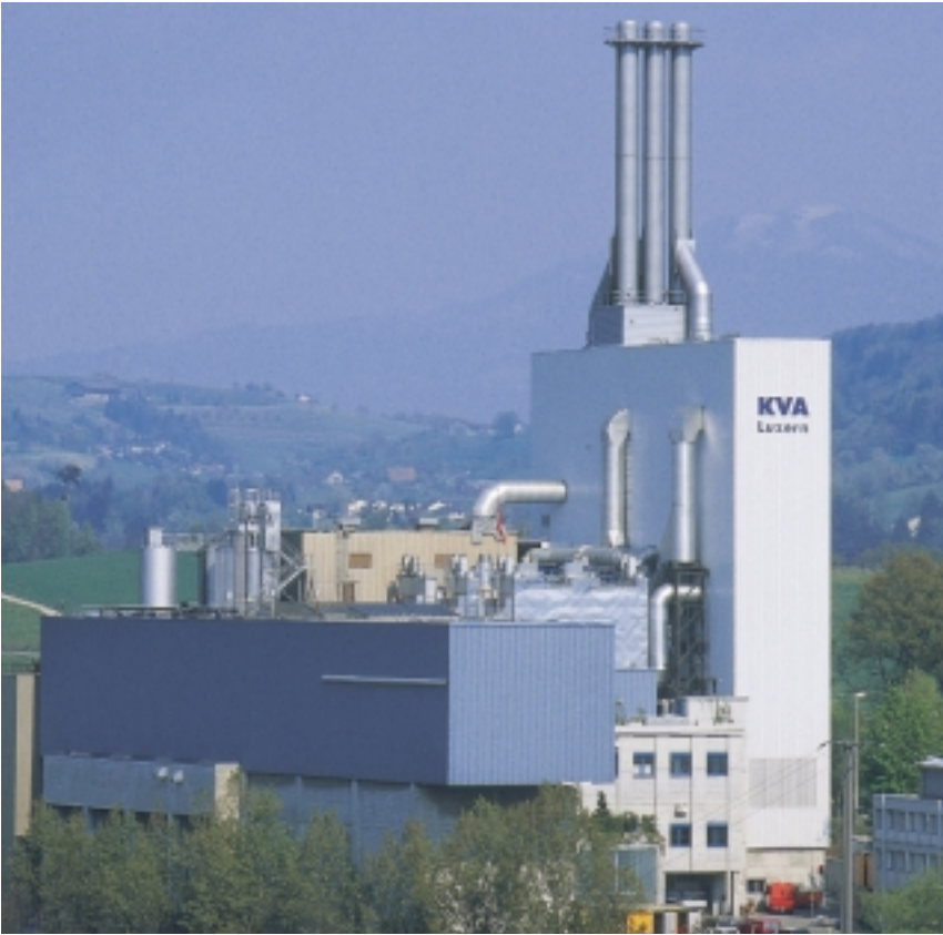
'Lucerne 2000' waste-to-energy power plant with new Air Pollution Control system from ABB Fläkt
