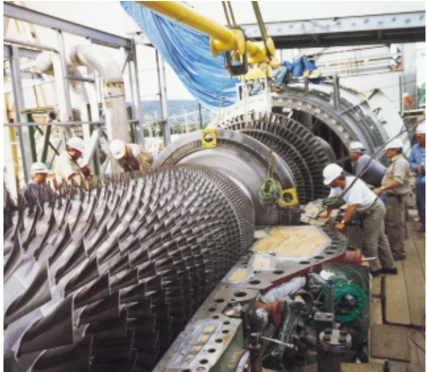
GT24 gas turbine being installed in the Gilbert power plant, New Jersey, USA 5
