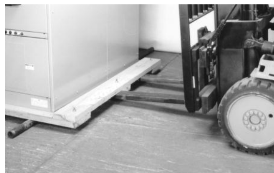
Fig. 2.7 Placement of rollers under shipping skid
