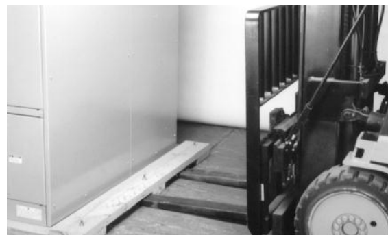
Fig. 2.6 Placing forklift tines under equipment shipping skid
