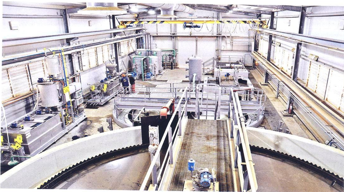
Figure 3: Hangar H-101 (Hassi R'Mel)
