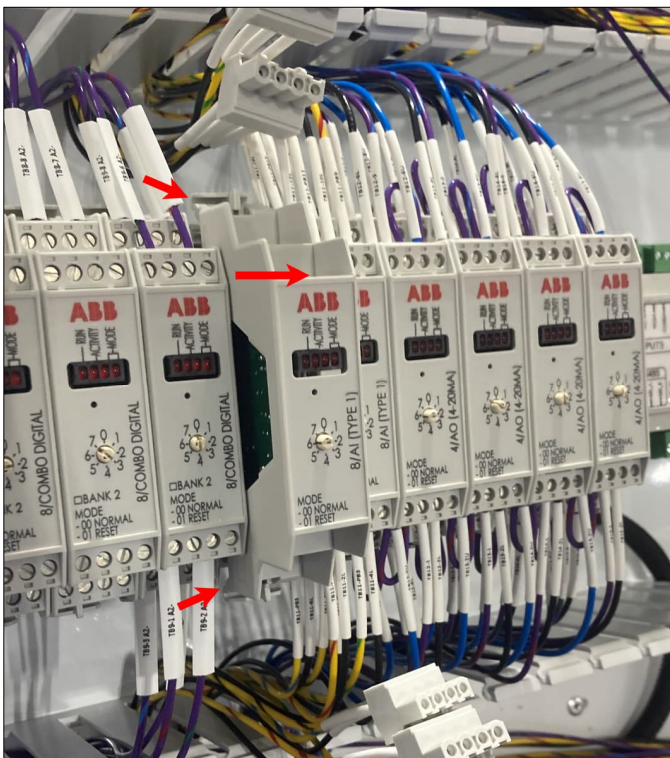
Figure 3-5: Remove module circuit board
