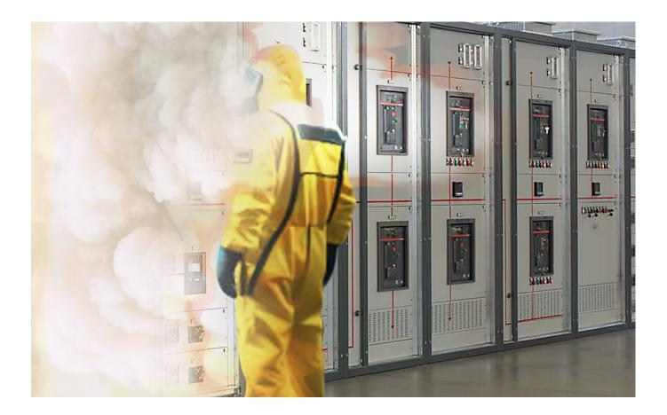
An arc flash is a dangerous condition associated with the release of energy caused by an electrical arc.
