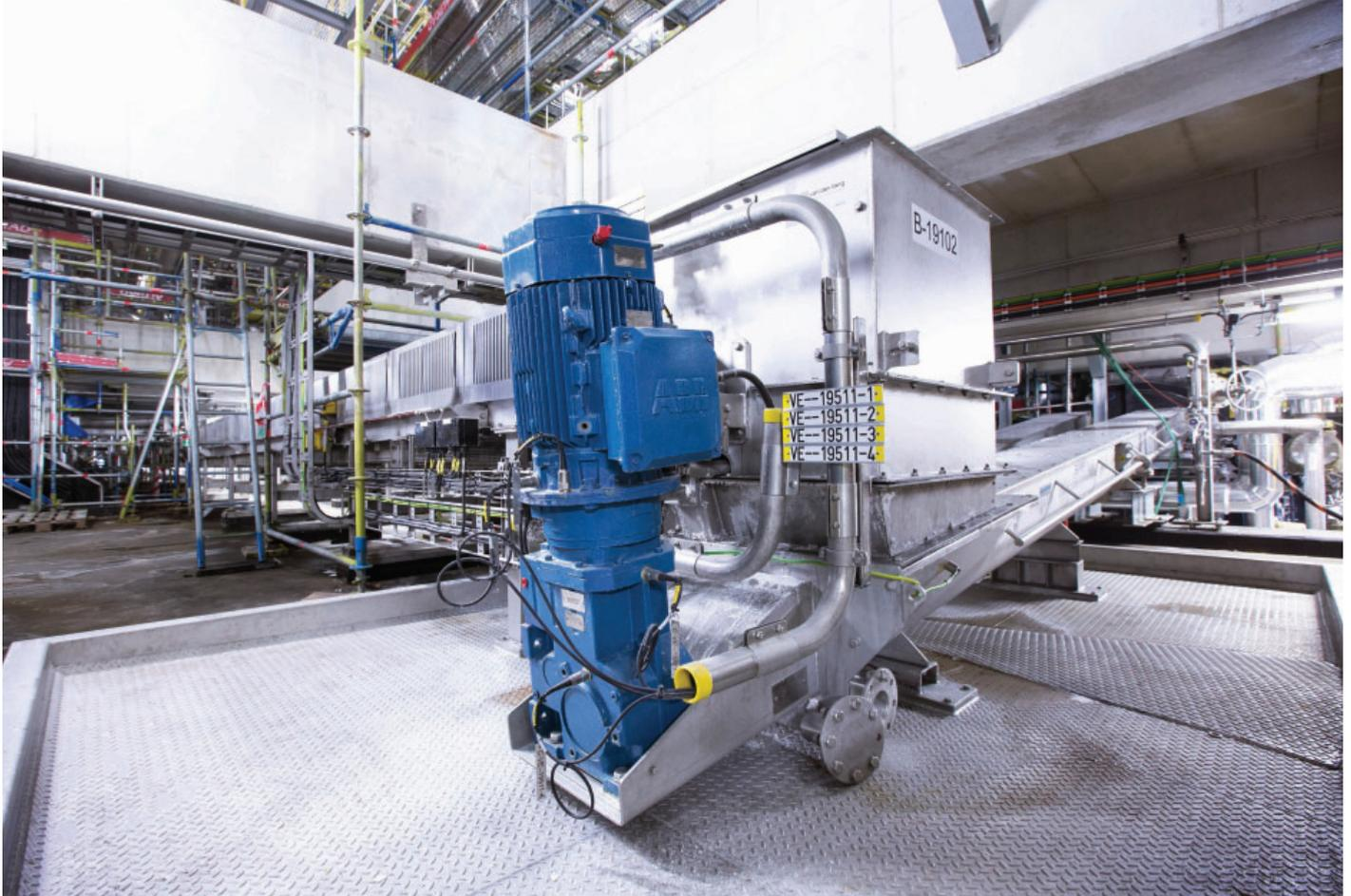
Installed on one of the 17 screw conveyors at the DSM plant, this Dodge Quantis right-angle bevel (RHB) gear reducer and ABB low voltage IEC motor creates a highly reliable drive train package.
