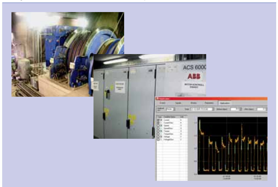
3 DriveMonitor – Analyzing the system’s heartbeat. Drive information can be utilized on various diagnostic levels – from the converter unit to the process section
