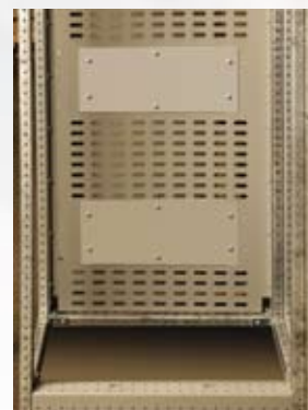
Rear cable area.
