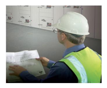
Condition-based maintenance is not only looking at actual data, it analyses the information as part of onsite condition monitoring packages like the MService for MNS iS. The MService system collects detailed information from the switchgear installation. This information not only contains electrical parameter, it also includes maintenance values such as contact temperatures or insertion cycles of a functional unit.
