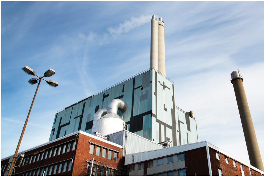
The Heleneholm plant in Malmö where E.ON has opted to use Pluto D45 for its safety solutions.
