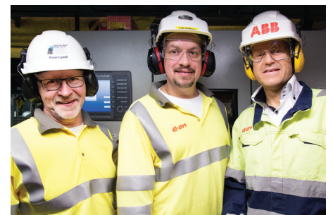
Peter Lysell from Industri-Teknik Bengt Fridh, André Strömberg from E.ON, Heleneholm plant and Anders Dieterle from ABB, in front of an equipment cabinet where Pluto is installed.
