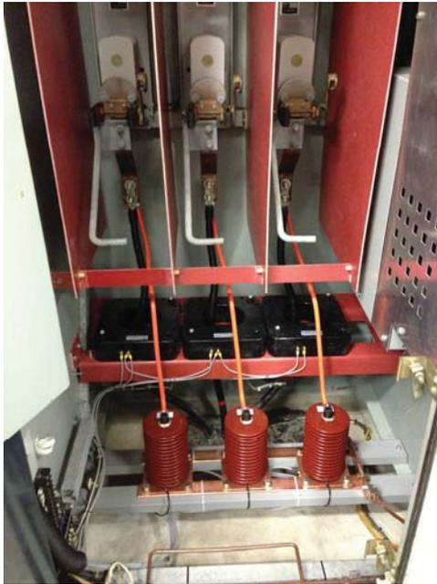
Fig. 14 An example of a 3 pole HSGS retrofit
