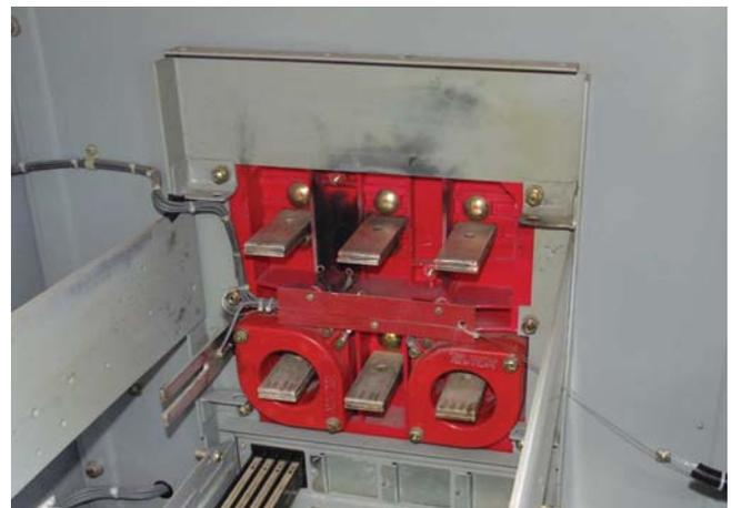
Fig. 10 Photo of damage to feeder compartment after arc fault with HSGS protection.
