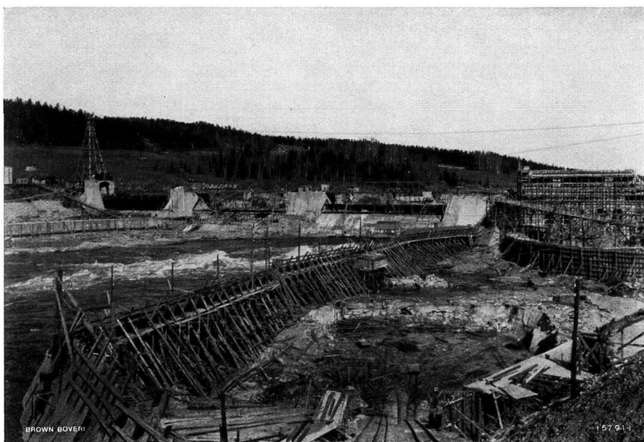
Fig. 3. — Condition of the work on March 26, 1921.
