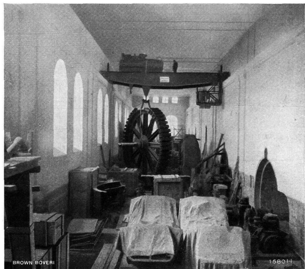
Fig. 13. — Progress made in erection up to October 14, 1921.
