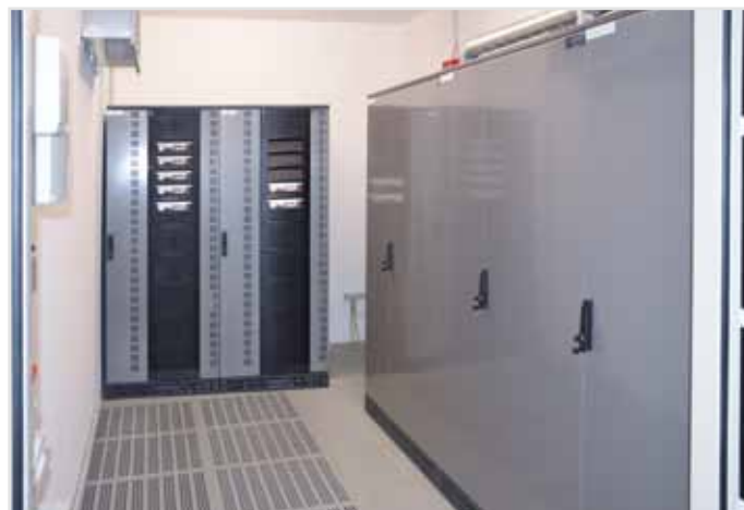
Newave Conceptpower DPA with 400 kW and 10 minute autonomy across 12 m 2
