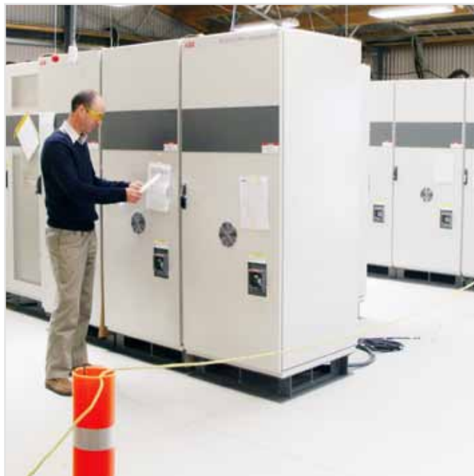
Power Protection Sales Manager, Andrew Hiscock, analysing the data sheet before the PCS100 UPS-Is are tested
