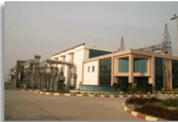
Substation Control Centre, Maharani Bagh, New Delhi
