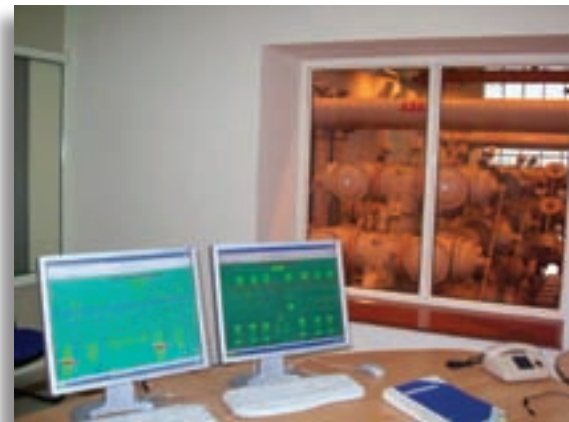
IEC 61850 Substation Automation System
