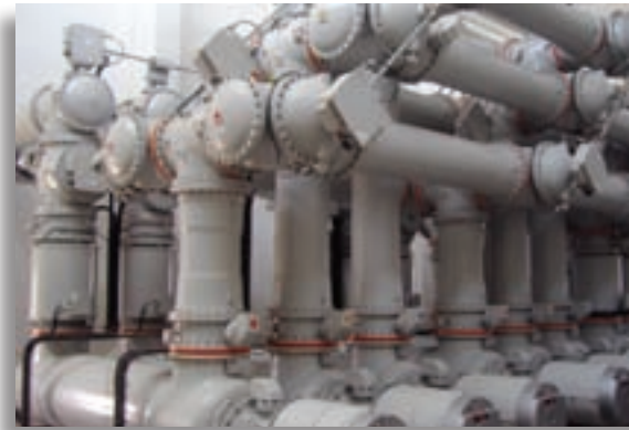
400kV Gas Insulated Switchgear
