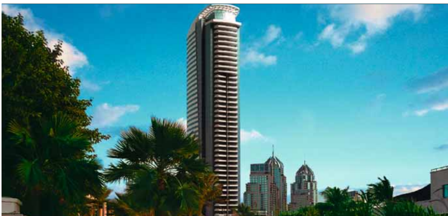
4 Le Rêve Tower in Dubai
