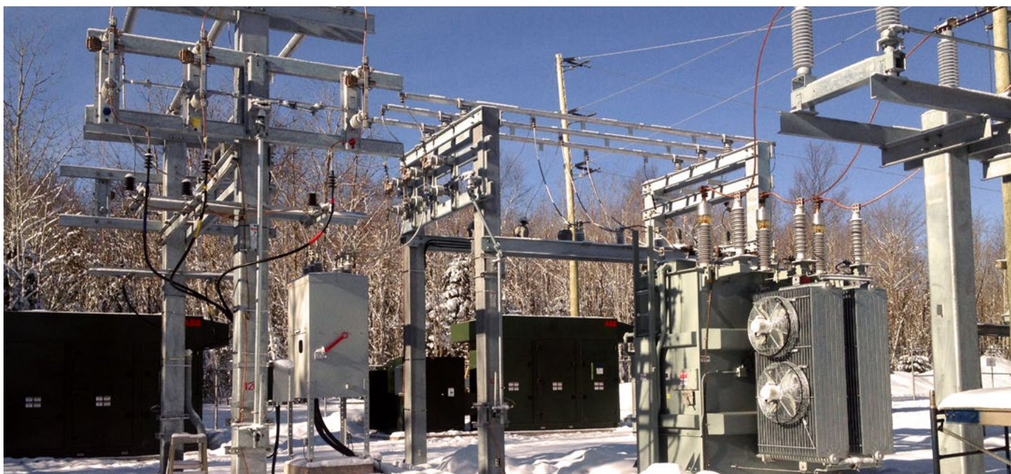
VArPro STATCOM installation at a substation in the Canadian Maritimes to support a growing power generation profile
