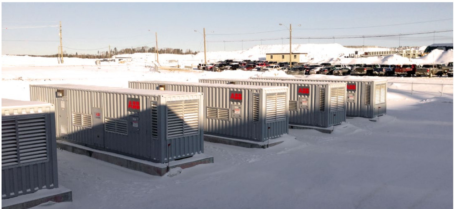
A line up of ABB's containerized STATCOMs in operation during Ontario's winter months.
