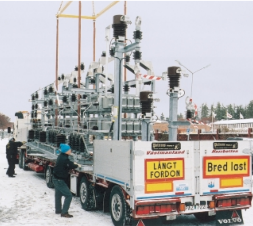
RSVC TSC module ready for transport
