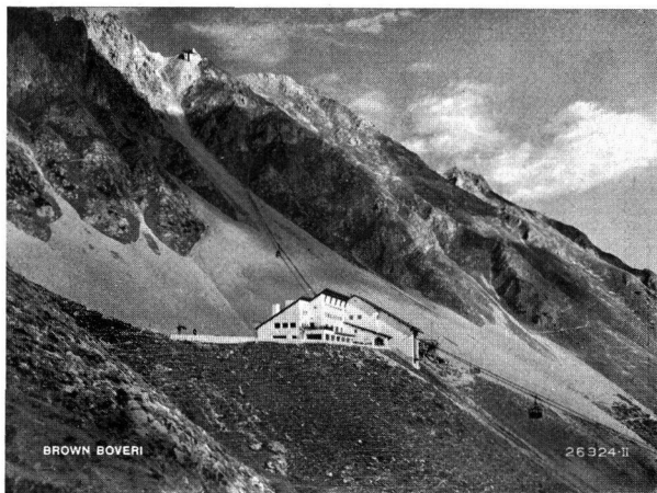
Fig. 1. — Intermediate station on the Nordketten Railway near Innsbruck.
