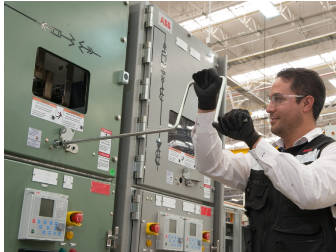
Fig. 17 Insertion of the contactor
