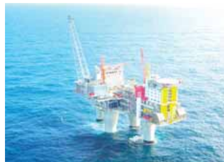
An offshore platform
