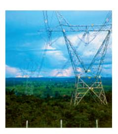
Without these, additional transmission lines would have been necessary to transmit an equal amount of energy. Shunt reactor compensation was also inserted at intervals along the line to maintain satisfactory system conditions over the full range of power transfer.
