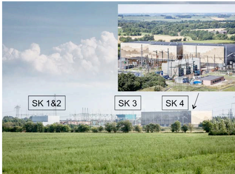
Figure 5. Skagerrak Converter Station, Tjele Terminal
