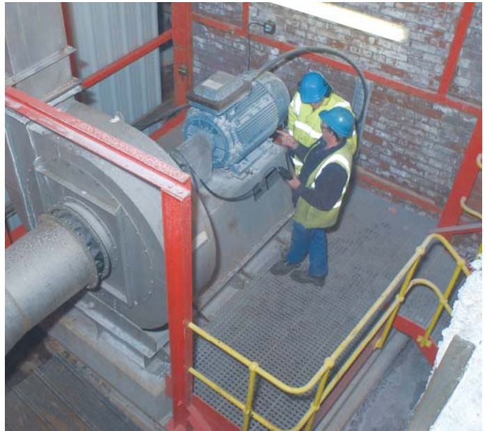
132 kW motor, coupled to an ABB industrial drive, saves over 1.6 GWh per year compared to the old 337 kW motor.
