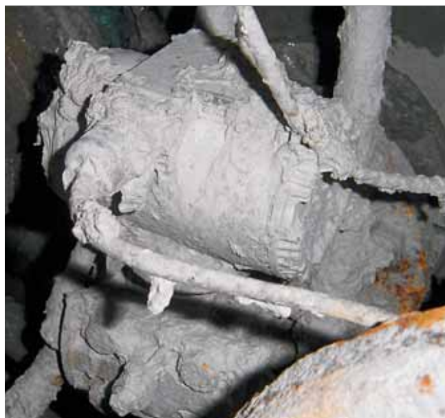
1 Differential pressure transmitter in a harsh environment: access for maintenance is hard
