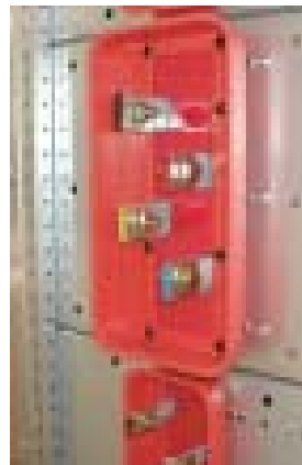
Outgoing terminals with boot retainer
