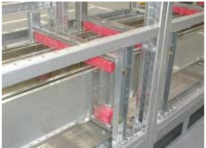
4000A main Busbars
