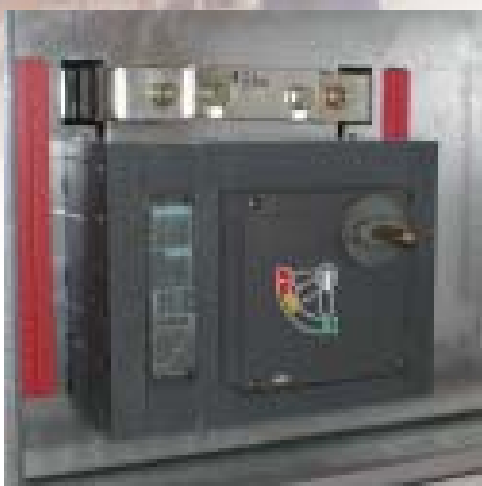
MCCB in cassette mounted in switchboard
