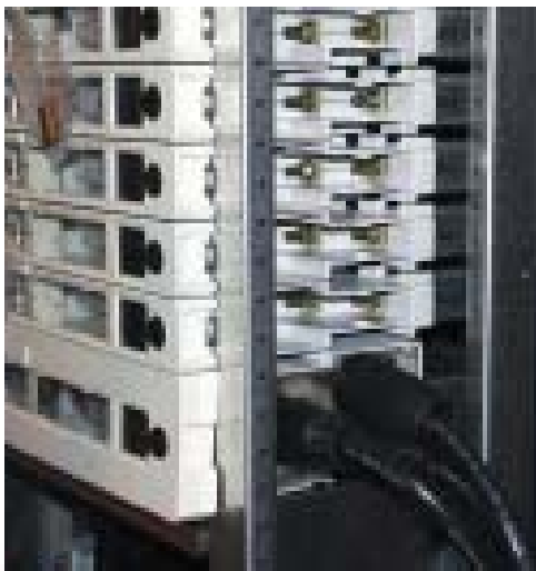
Slimline Switchfuse with outgoing cables
