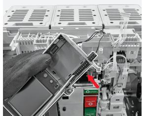
By means of the torx key unscrew the screw fixing the plug to the trip unit.
