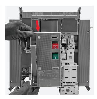
By means of the cross screwdriver unscrew the 2 + 2 screws fixing the left and the right shields to the circuit breaker.
