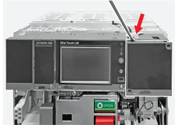
**38** By means of the cutter start removing the label located on the Ekip measuring blind module and by means of the pliers complete the removal operation.
