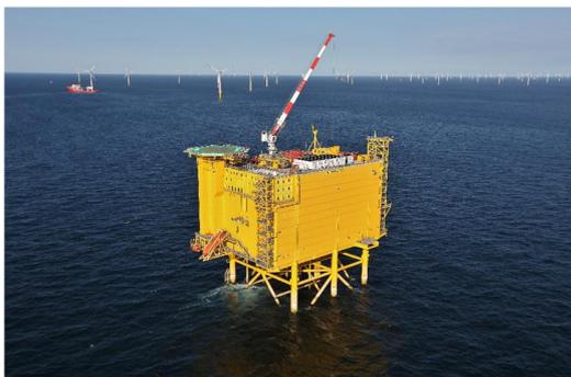
Figure 9 The DolWin1 grid connection can integrate 800 MW of offshore wind power around 75 kilometers off the German coast, enough to supply around one million households with clean energy
