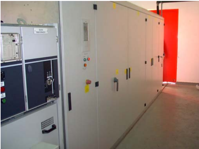
Fig. 7 (c) Frequency Converter enclosure
