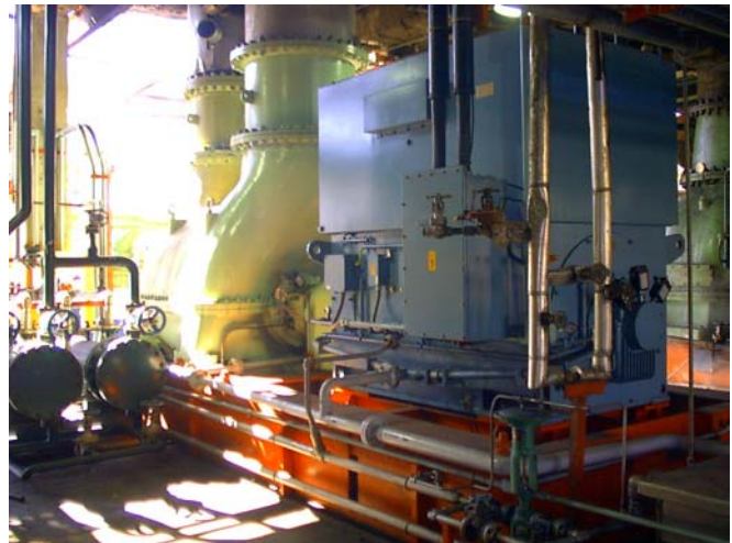
Fig. 7 (a) Drive Motor Installation
