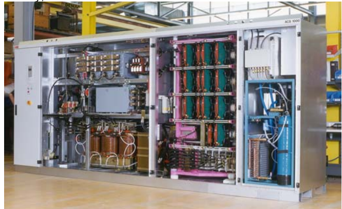
Fig. 4: Water cooled frequency converter 1: Control 2: Output Filter and DC-link components 3: Rectifier and Inverter stacks 4: Water cooling unit
