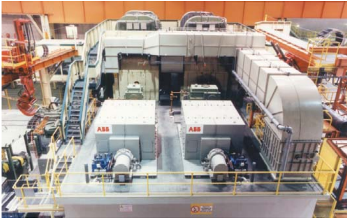
Fig. 2 Drive side, showing AC main drive motors
