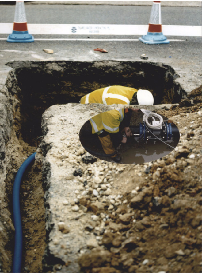
Underground Installation of MagMaster
