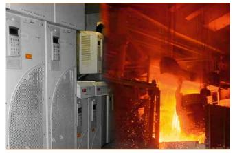
significant advantage of DTC is that it can achieve full torque at zero speed without any feedback device. It controls torque with an accuracy of one percent from zero speed through base speed without encoder feedback<sup>2</sup>.
