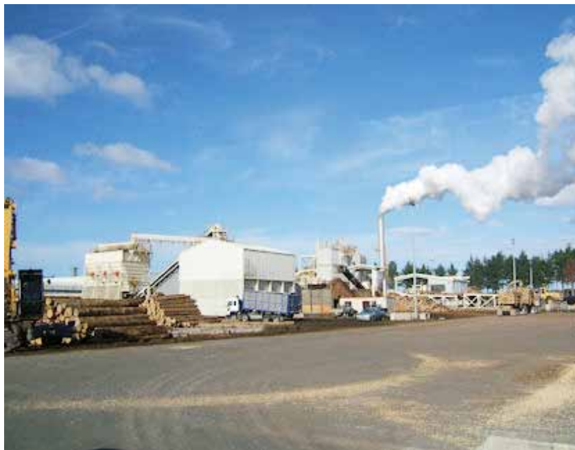
Carter Holt Harvey's LVL Mill in Marsden Point
