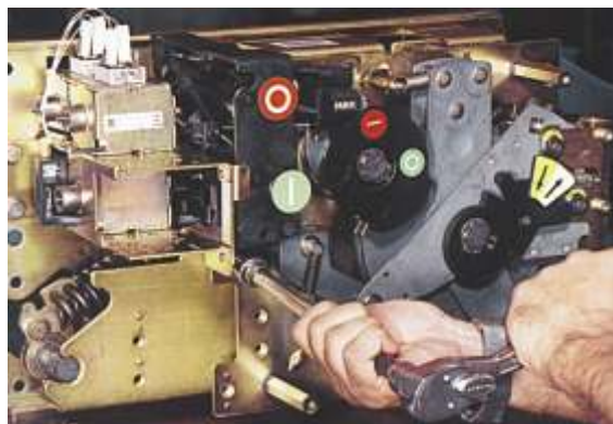
Unscrew the fixing screw of the release group mount
