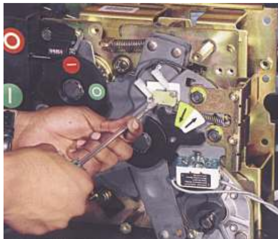
Unscrew the microswitch fixing screws
