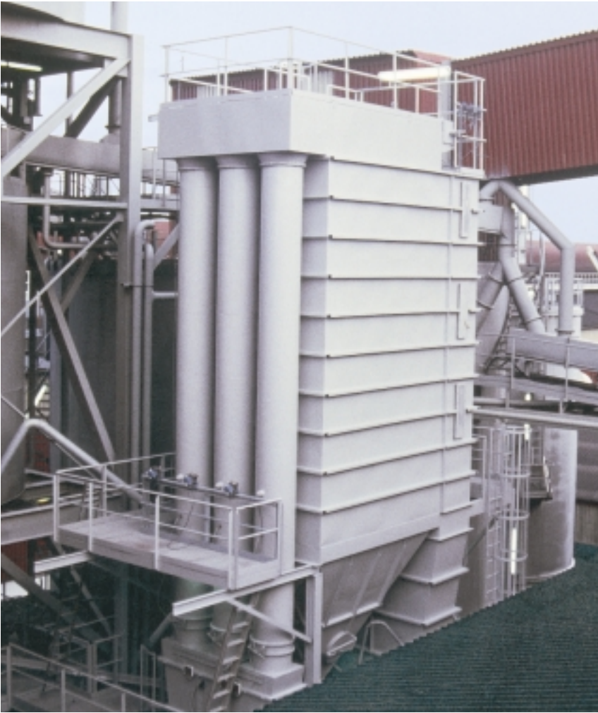
Pilot plant installed in a prebake smelter
