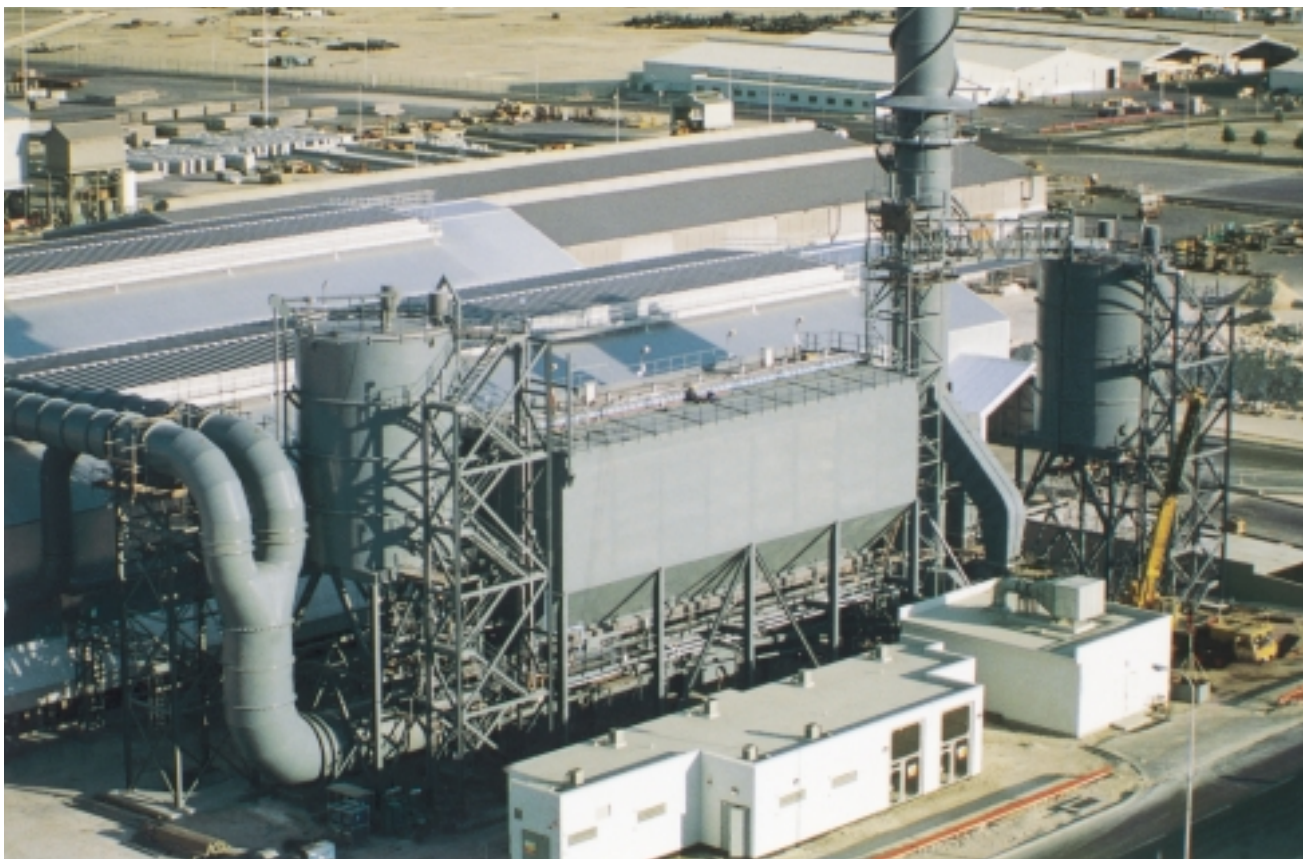
Full-size dry scrubber of ABBART design at the ALBA aluminium plant in Bahrain. The scrubber went on line in March 1997.
