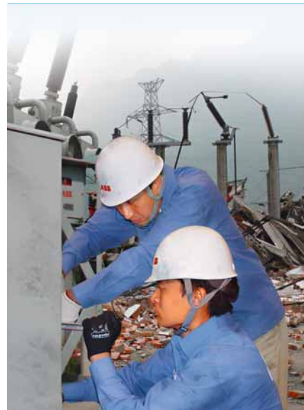
4 ABB engineers repair damaged HV breakers at Mianyang Power Supply after the massive Wenchuan earthquake in Sichuan.
