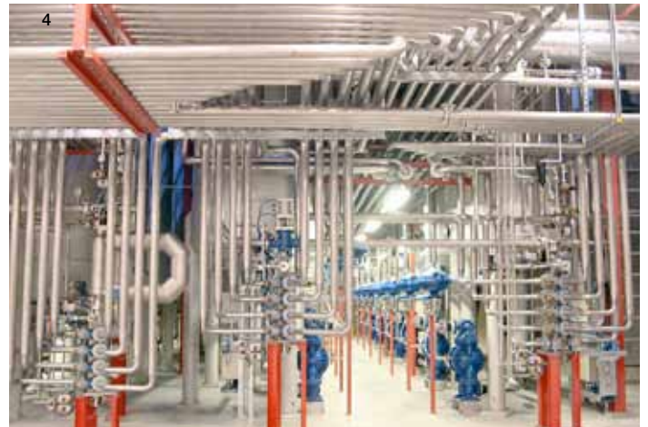
1 Powder conveying screws on metering hopper | 2 Piggable manifold with pig loading stations | 3 Storage tanks in Atex area with operator terminal | 4 Piggable collectors to precisely dose liquid materials through mass-flow meters
