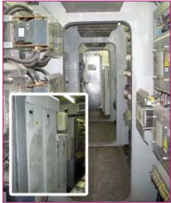
Electric room inside the gantry.
