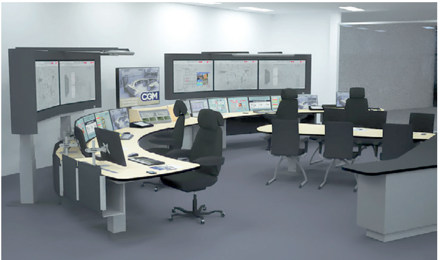
Fig 2. An ergonomically-planned control room with optimally positioned consoles and screens helps operators monitor processes and detect events.
