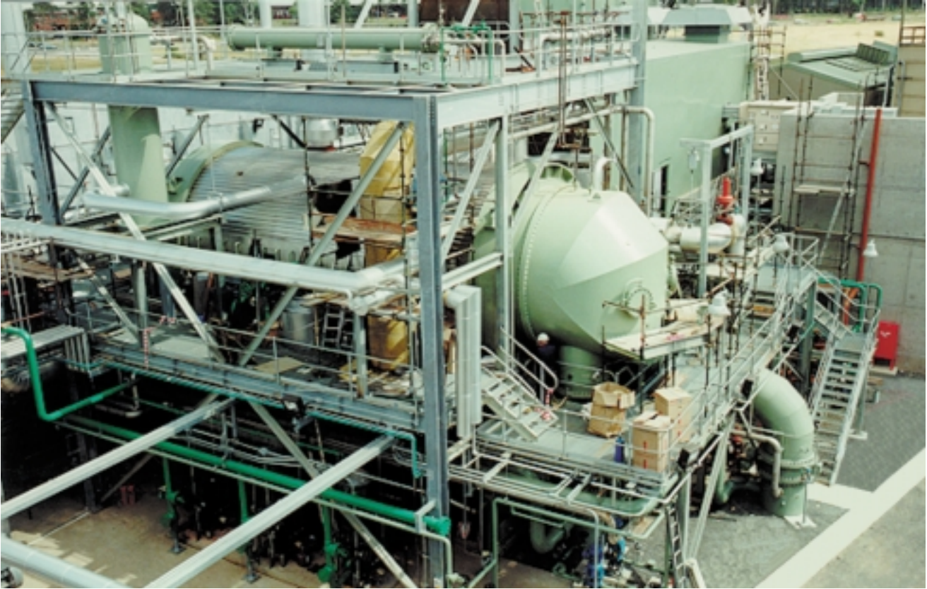
CB/A steam condenser in the 180-MW combined cycle power station of Smithfield Energy Facility, Australia
