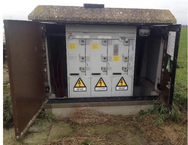
Figure 1. SafeRing AirPlus CCV switchgear installed at CSS 3 in Zeewolde, Netherlands.
