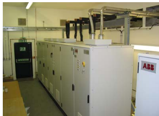
Figure 14: Indoor installed STATCOM converter units
