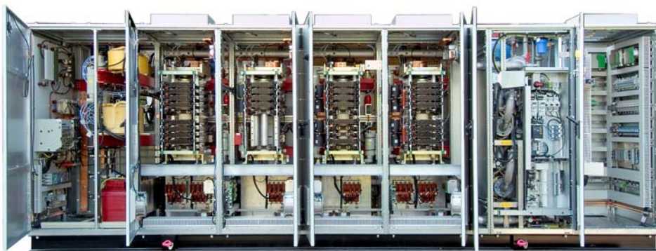
Figure 10: View of a PCS 6000 STATCOM converter cabinet
