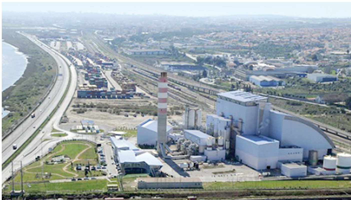
One-fifth of Portugal's waste is processed and converted into electricity at the Valorsul waste-to-energy plant, Portugal
