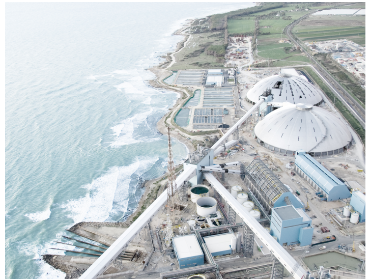
Figure 3: Clean coal-fired power plant
