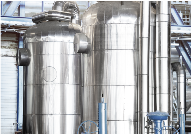
Figure 1: Clean coal power plant boiler (water condenser)
