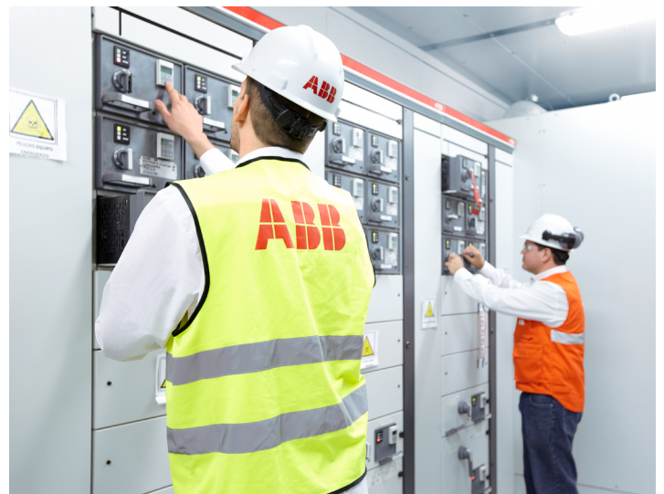
Figure 2: Variable Frequency Drives (VFDs)
